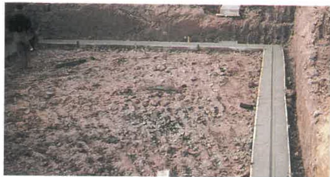
Fig. 26-13. When a concrete foundation is to be poured, the footing should be keyed. Key is formed by placing a wooden strip in the form during or immediately after the pour. (Portland Cement Association)
