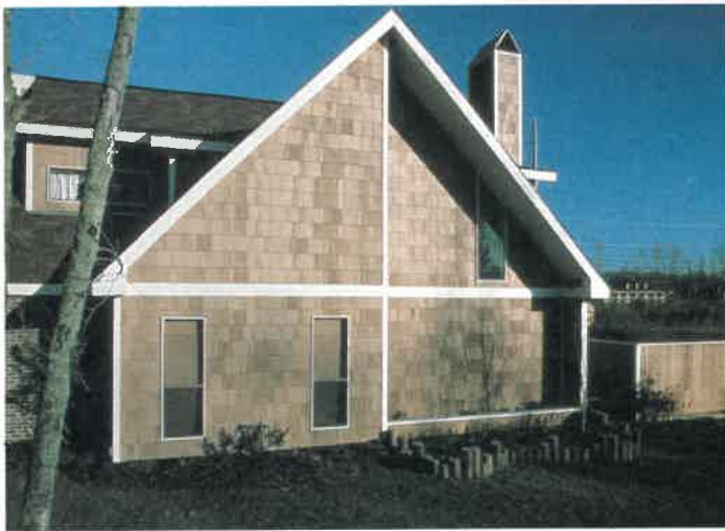
Fig. 29-30. Home sided in shingle panels manufactured from hardboard. Panels are made in 8 ft. and 16 ft. lengths. (Masonite Corp.)
