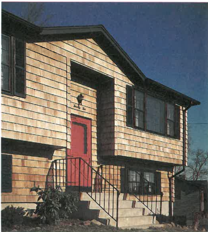
Fig. 29-28. Wood shingles form a durable and attractive exterior wall covering. (Shakertown Corp.)
