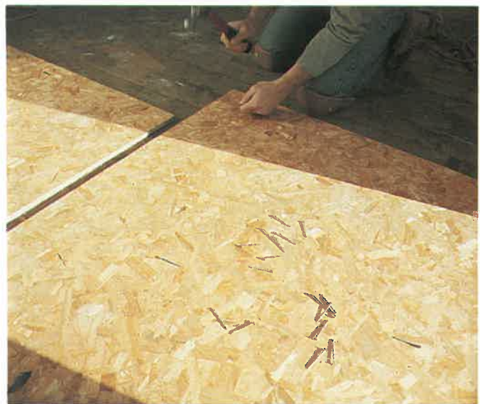
Fig. 35-45. Waferboard panel products include sheathing, soffits, and several other applications. (Georgia Pacific Corporation)
