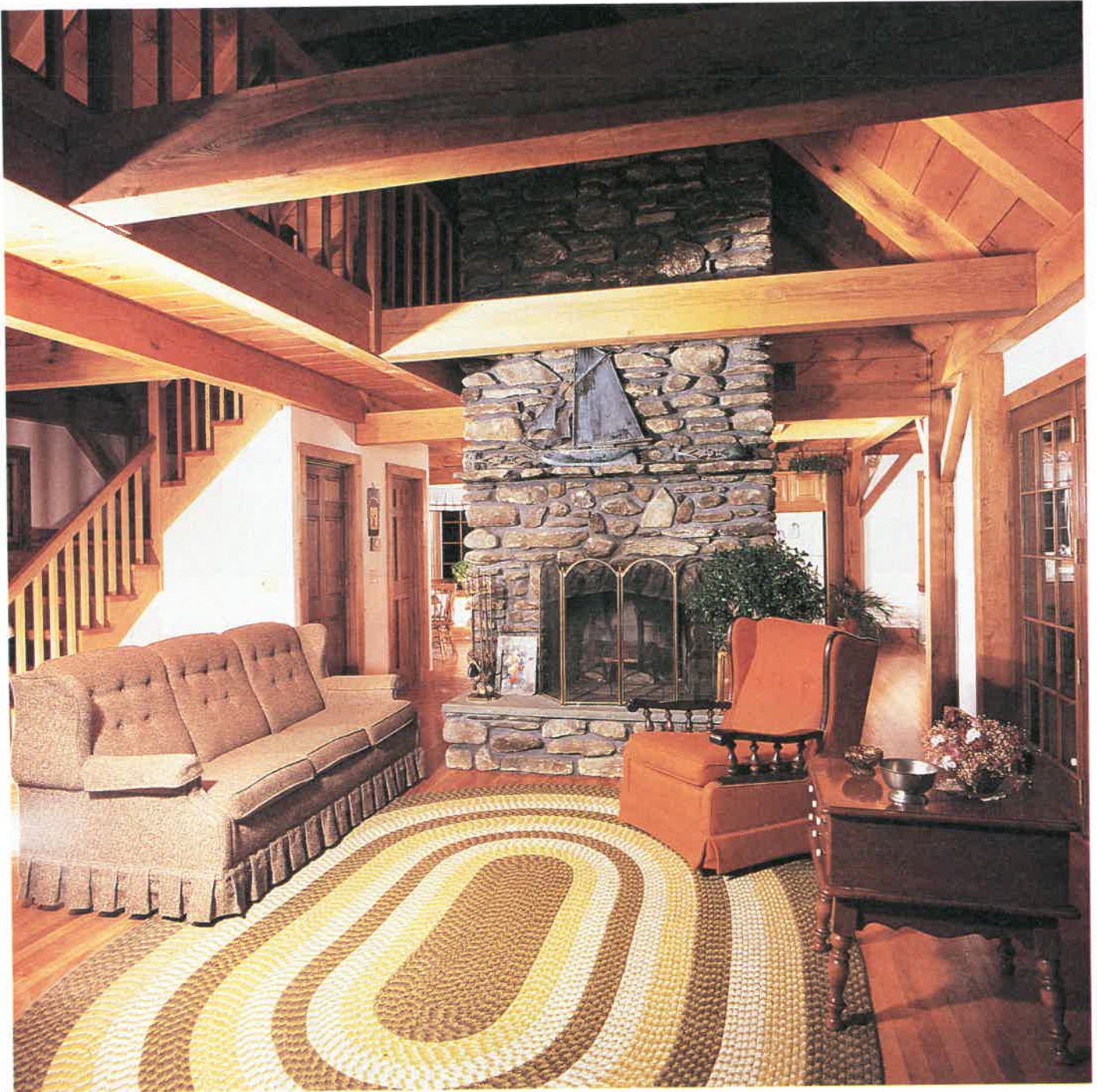
Post-and-beam construction opens up interior space by providing large spans that do not need support walls or posts. (E.F. Bufton and Son)
