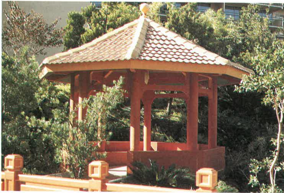
Fig. 28-42. This durable clay tile roof will withstand high winds, rain, and severe weather.
