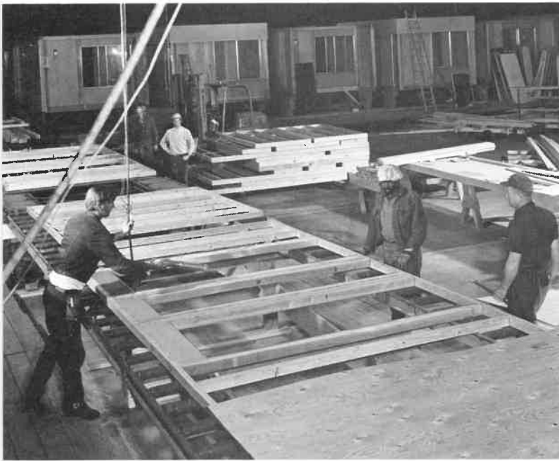
Fig. 31-17. Wall panels under construction on a production line.
