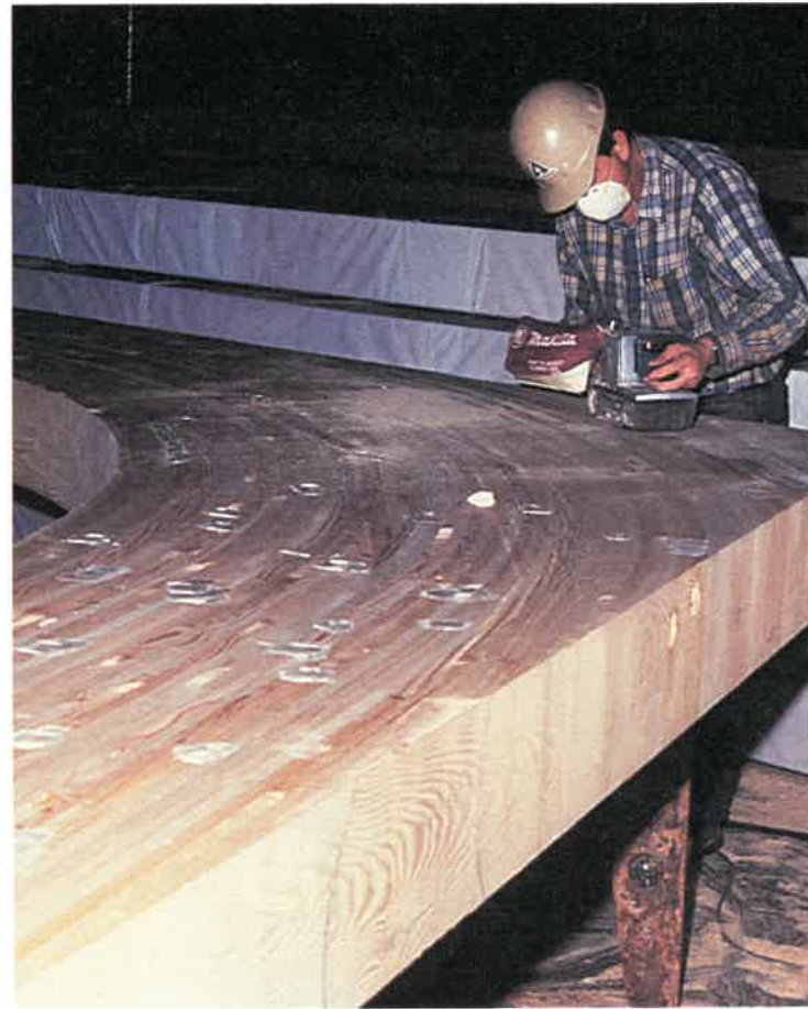
Fig. 23-20. Final sanding and inspection of giant laminate arches. After coats of finish are applied, they will be wrapped in a waterproof covering for shipment to the construction site. (John Walker)
