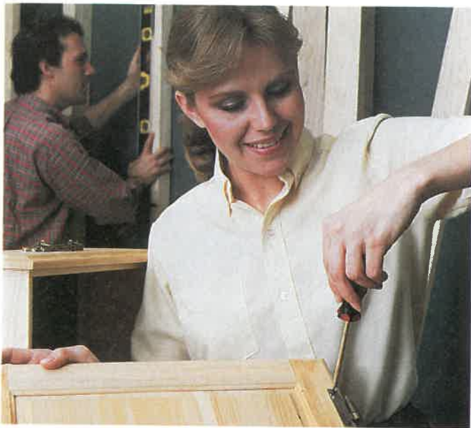
Fig. 12-9. Prefitted hardware being removed before finish is applied. (The Stanley Works)
