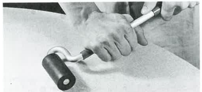
Fig. 24-9. Applying pressure to the laminate with a hand roller. Press down hard with both hands.
