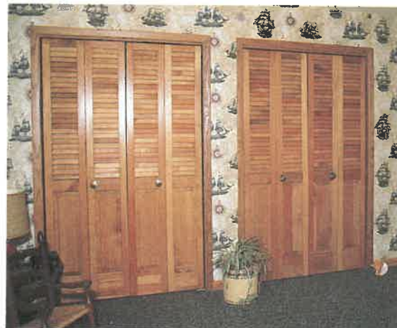
Fig. 30-28. Bi-fold doors are often used to close off closet space. (C.E. Morgan)
