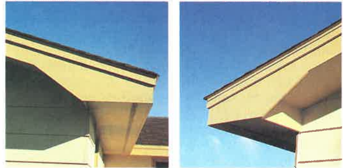
Fig. 29-24. Two views of a completed cornice and rake. Note continuous vent system in soffit. (Dickinson Homes, Inc.)
