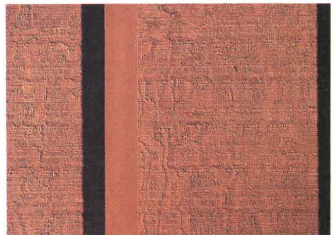
Fig. 29-27. Textured plywood panels provide the basic siding material in this photo. Narrow strips of wood were added to cover the joints and add decoration. (American Plywood Association)
