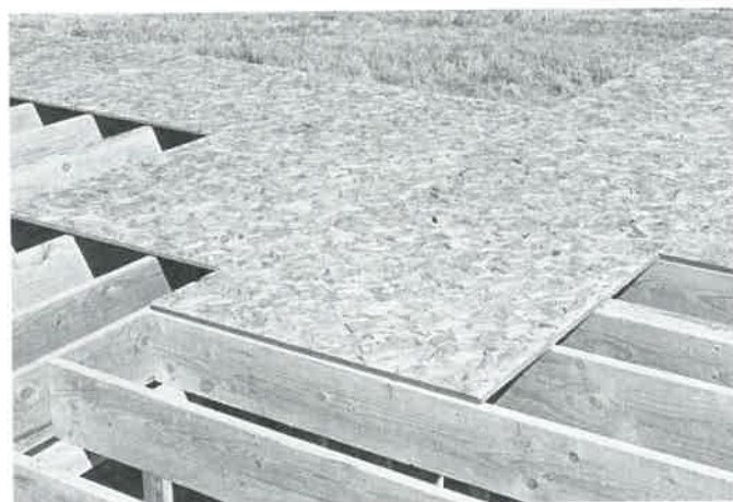
Fig. 27-33. Waferboard panels are engineered and approved for use in subflooring. The same application methods are used as for plywood. For non-textile resilient floor applications a 1/4 in. underlayment is recommended. (Louisiana-Pacific Corp.)
