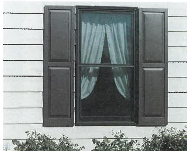
Fig. 29-1. Typical double-hung window with screen in place. Nonfunctional shutters have been added for overall appearance. (Caradco Corp.)
