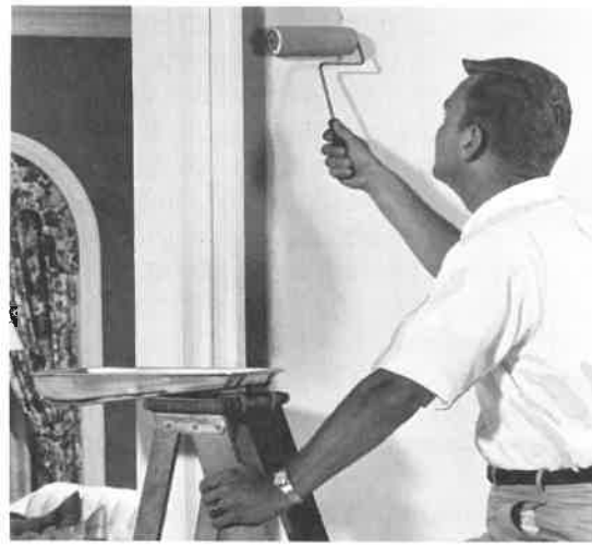
Fig. 12-33. Using roller to apply latex wall paint. (Sherwin-Williams Co.)
