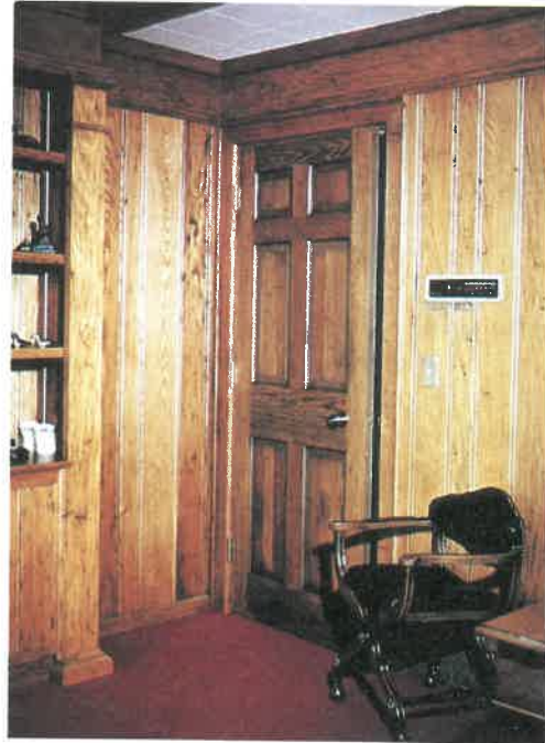
Fig. 30-27. Standard interior panel door. In good residential planning, passage doors are located so they will swing open (90 deg.) against another wall, as shown. (C.E. Morgan)
