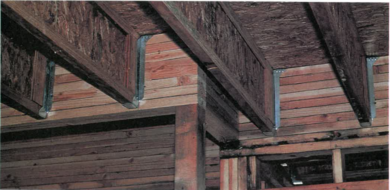
The ceiling joists in this modern frame structure are engineered wood I-joists and the supporting beams are glue laminated beams. (American Plywood Association)
