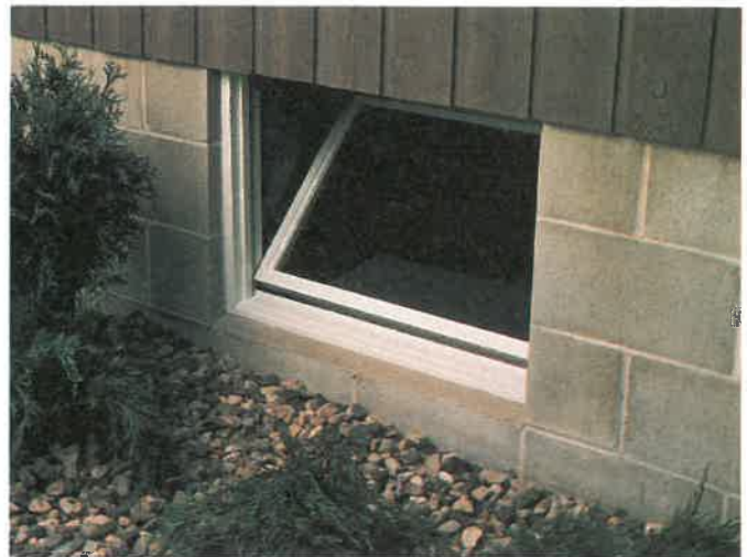
Fig. 26-27. Installing windows in basement walls. Top. Detail of basement window unit that can be placed in a concrete or masonry foundation wall. Bottom. Unit installed. (Andersen Corp.)
