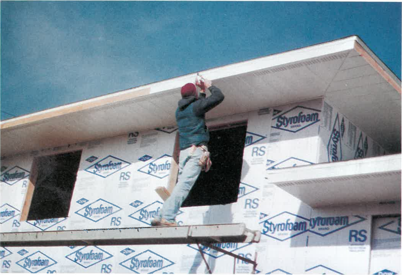
Installing the fascia of a prefabricated soffit system.
