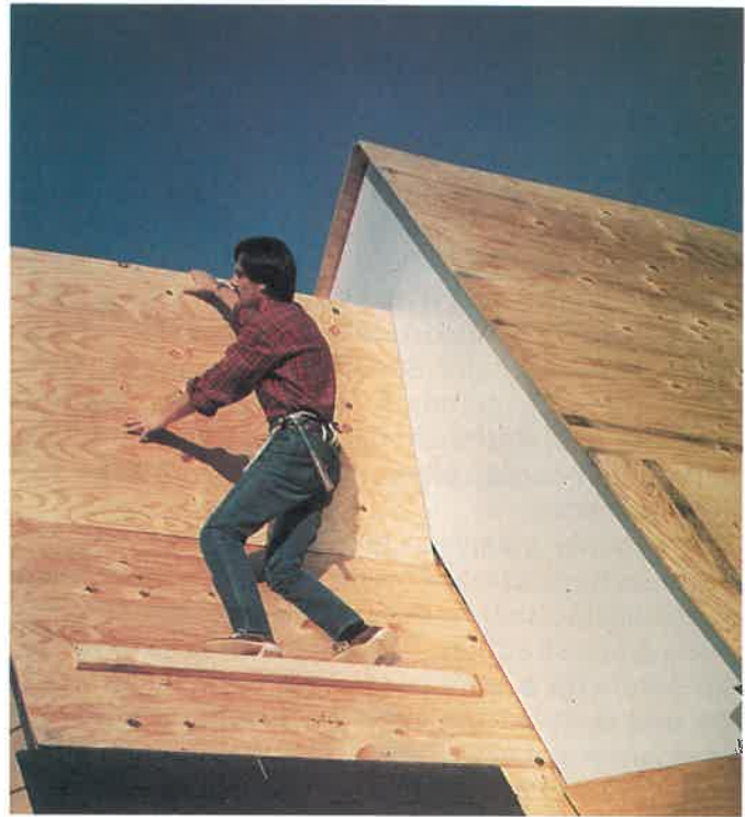
Fig. 36-12. Carpenter installing roof sheathing on a modern home. The work is physically demanding, but provides a sense of accomplishment when completed. (Georgia Pacific Corporation)
