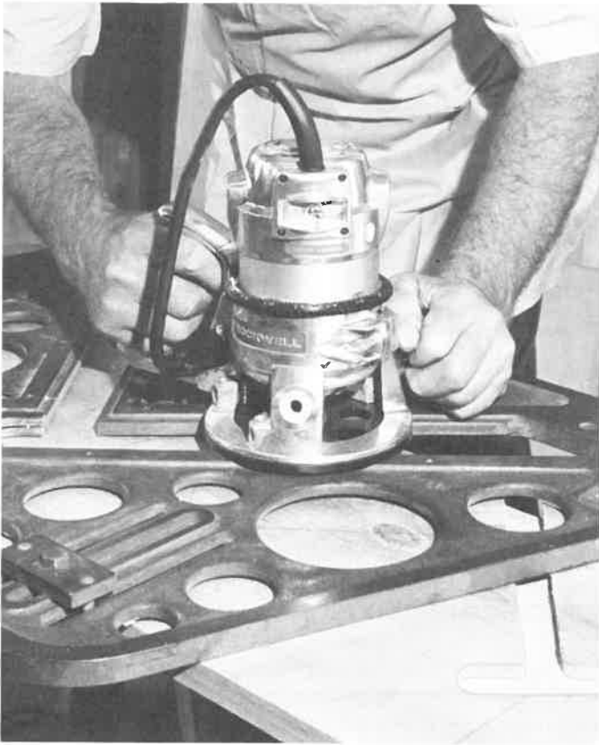
Fig. 18-20. Heavy-duty routers and stair templates are used to cut housed stringer. Stair treads and risers will be assembled in the grooves.
