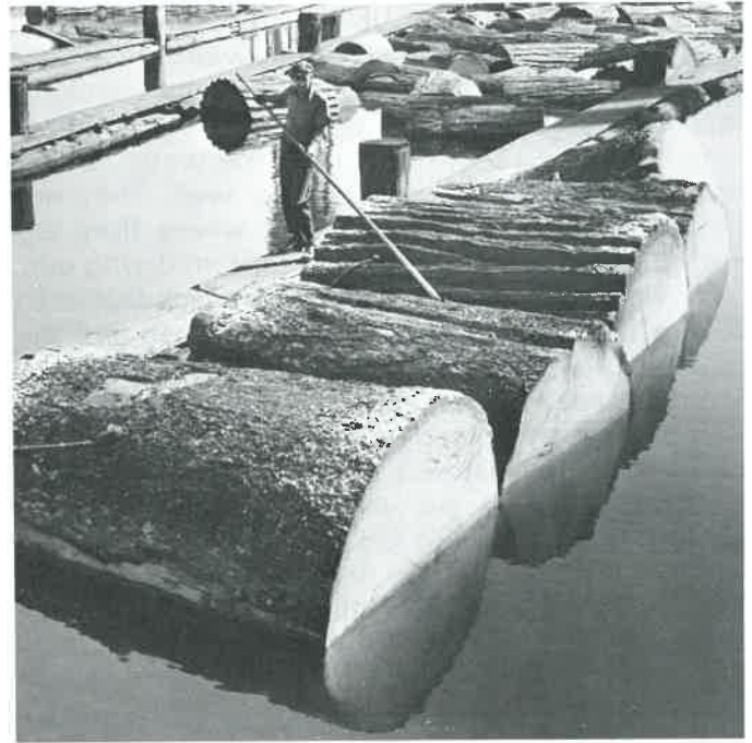
Fig. 35-27. Selected "peeler" logs, cut from the lower portion of the tree, are used for plywood. (American Plywood Association)
