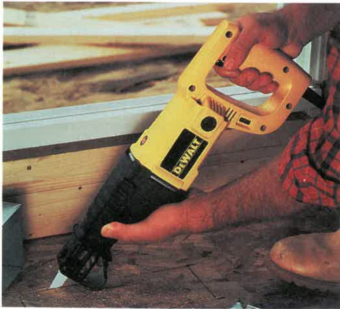
Fig. 15-40. Using the reciprocating saw to rough-in an opening. (DeWalt)
