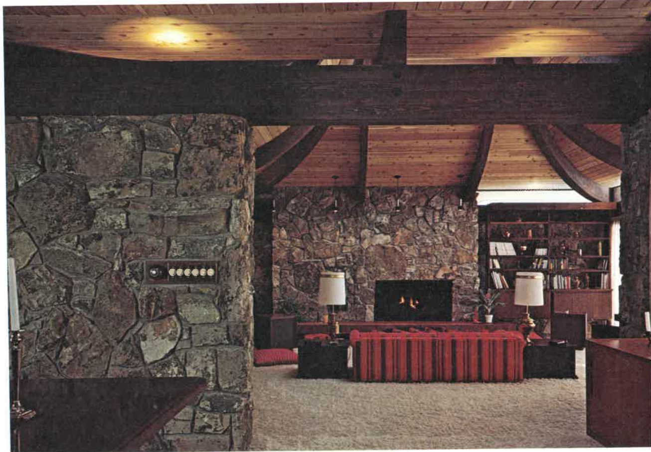
Two views of a dining/living room combination that takes advantage of the large, open space provided by both curved and straight laminated beams. (Potlatch Corp.)
