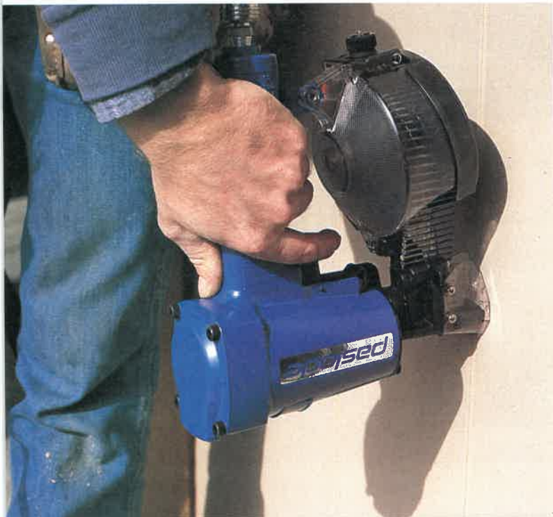
Fig. 10-30. Attaching a panel using a light duty air-powered brad nailer. (Paslode Co., Div. of Signode)
