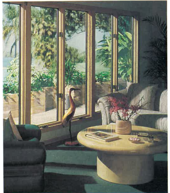
Fig. 29-3. Casement windows are hinged on the side and are operated with a hand crank.
