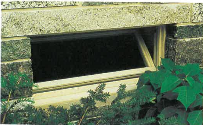
Fig. 29-5. Hopper window. (Andersen Corp.)
