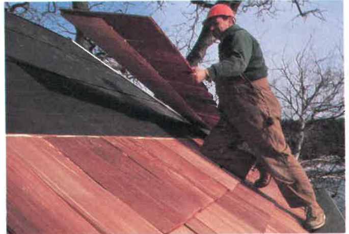
Fig. 28-40. Applying shingle panels to a roof. Panels are prefabricated in 8 ft. lengths. (Shakertown Corp.)
