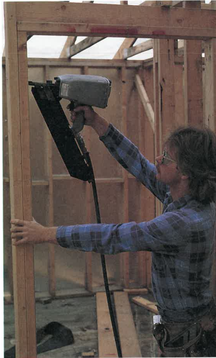
Top left. Engineered wood floor trusses used as floor frame. (Southern Forest Products Association) Bottom left. Pressure treated 2 x 6 southern yellow pine decking. (Southern Forest Products Association) Right. Using a power nailer to install a door trimmer. (Paslode Co., Div. of Signode)
