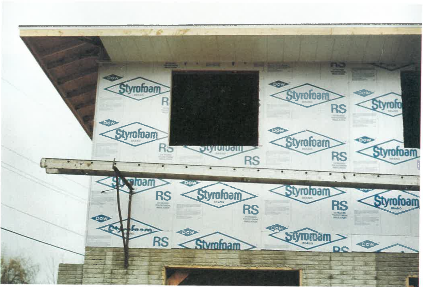
Rigid polystyrene foam sheathing. Panels are 1 in. thick and 96 in. long. They have an R-value of 5.50.
