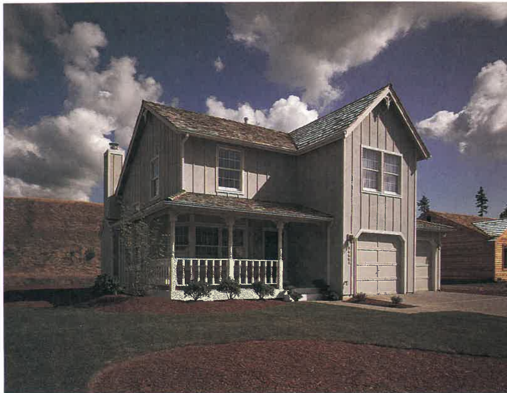
Roof design and roofing materials are important elements in the appearance and function of this structure. (American Plywood Association)
