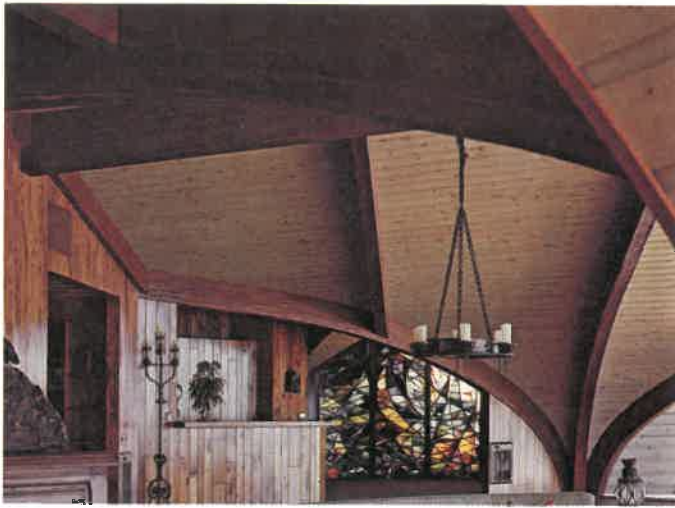
Fig. 23-14. The curved support beams of this modern structure are laminated beams. They provide great strength and freedom of design. (Potlatch Corp.)
