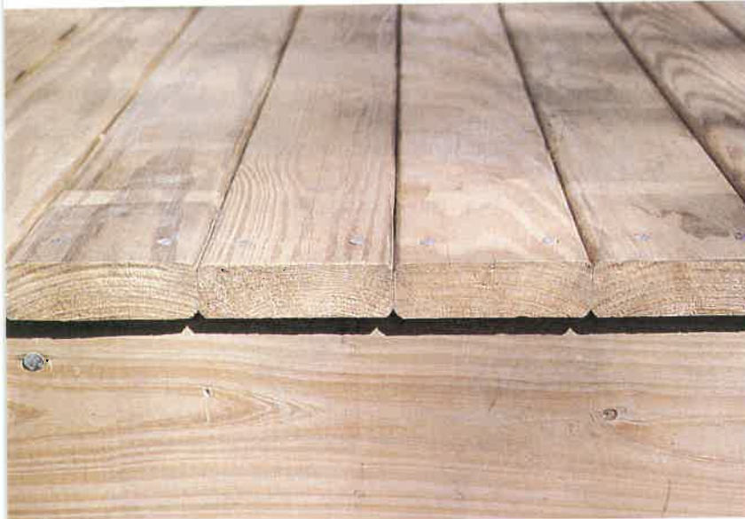
Top left. Engineered wood floor trusses used as floor frame. (Southern Forest Products Association) Bottom left. Pressure treated 2 x 6 southern yellow pine decking. (Southern Forest Products Association) Right. Using a power nailer to install a door trimmer. (Paslode Co., Div. of Signode)
