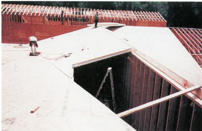
Insulated sandwich panels are being used to form the roof of this large home. (AFM Corporation)
