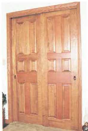
Fig. 30-29. Bypass doors used for closet space. The doors open from either side. (C.E. Morgan)
